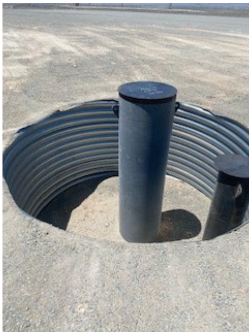
Figure 11: Conductor and mouse - as constructed.
