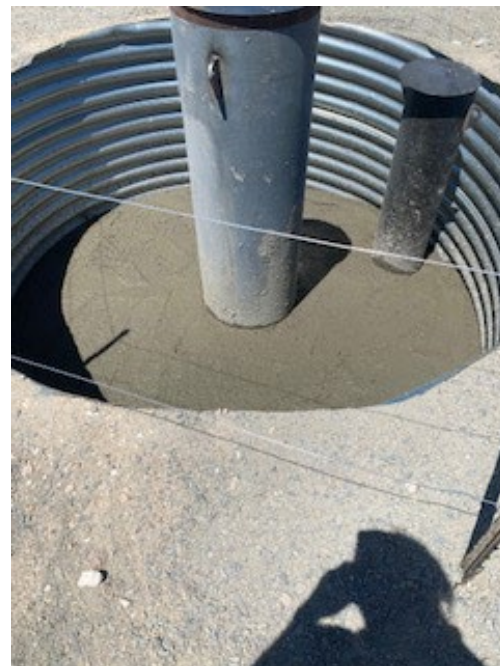
Figure 12: Lateral view, conductor and mouse hole.
