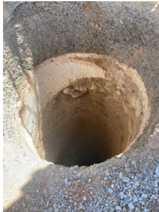
Figure 8: Conductor hole as drilled.
