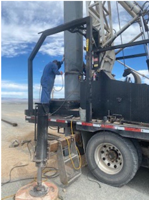
Figure 9: Conductor setting.
