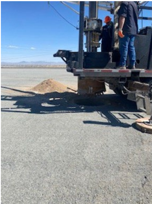
Figure 7: Drilling of conductor.
