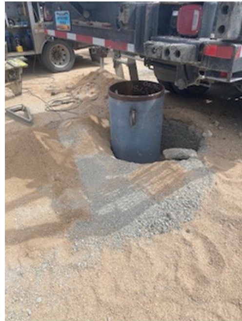
Figure 10: Conductor setting -cont.
